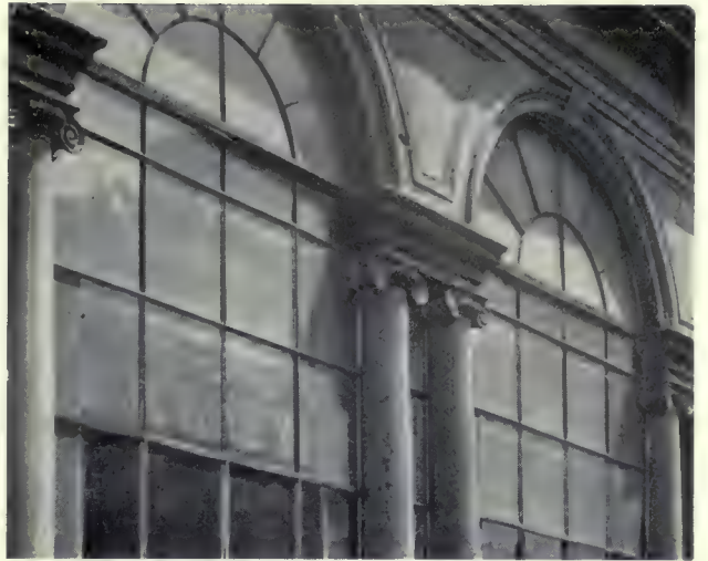
30. - Palazzo Borghese. Court, detail of capitals on northeast side.
